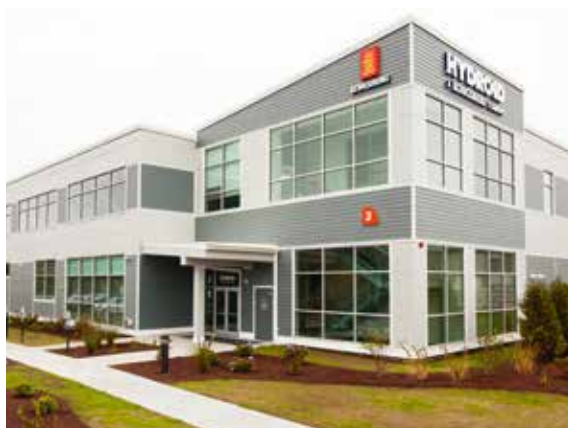
Right: From the energy centre for district heating, remote cooling and heat recovery at Kongsberg Technology Park.
