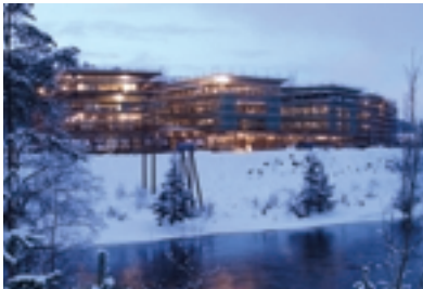
Kongsberg Simrad's new building, with room for about 550 new employees, is scheduled for completion in autumn 2001.
