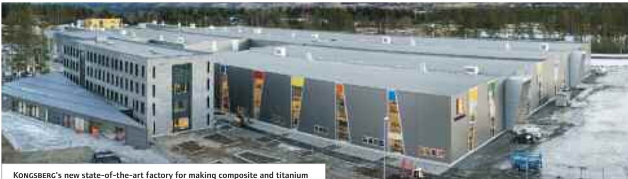
KONGSBERG's new state-of-the-art factory for making composite and titanium is one of the largest industrial buildings erected in Norway in recent years.
